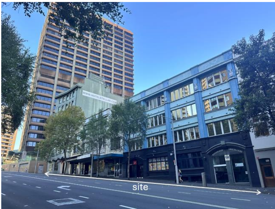
Figure 3: Subject row of warehouse buildings viewed from Wentworth Avenue, looking north-east
